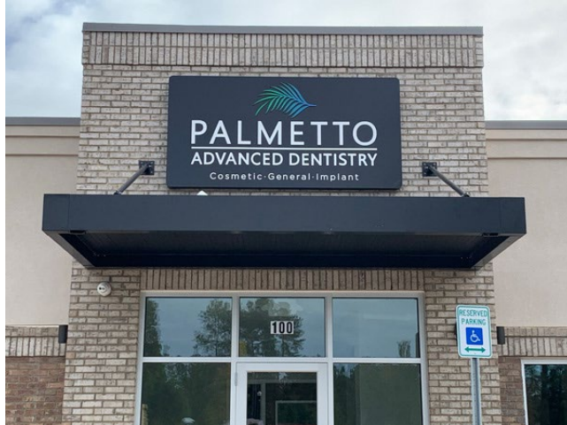
Figure X: Example of a wall sign
