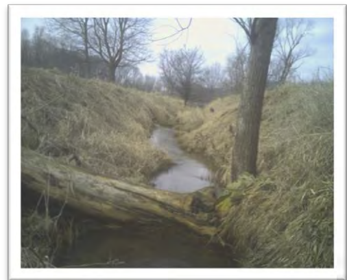
Photograph 6 (2-2-12). The ditch dug through the nature preserve is deeply entrenched.
