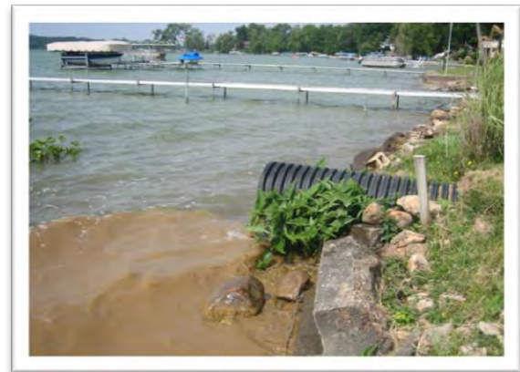
Photograph 7 (6-20-12). Agricultural drainage and associated pollutants drain to Oliver Lake from an adjacent field.
