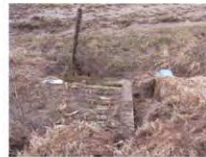
Oliver Lake-26 Facing down and north at inlet pipe to til...
