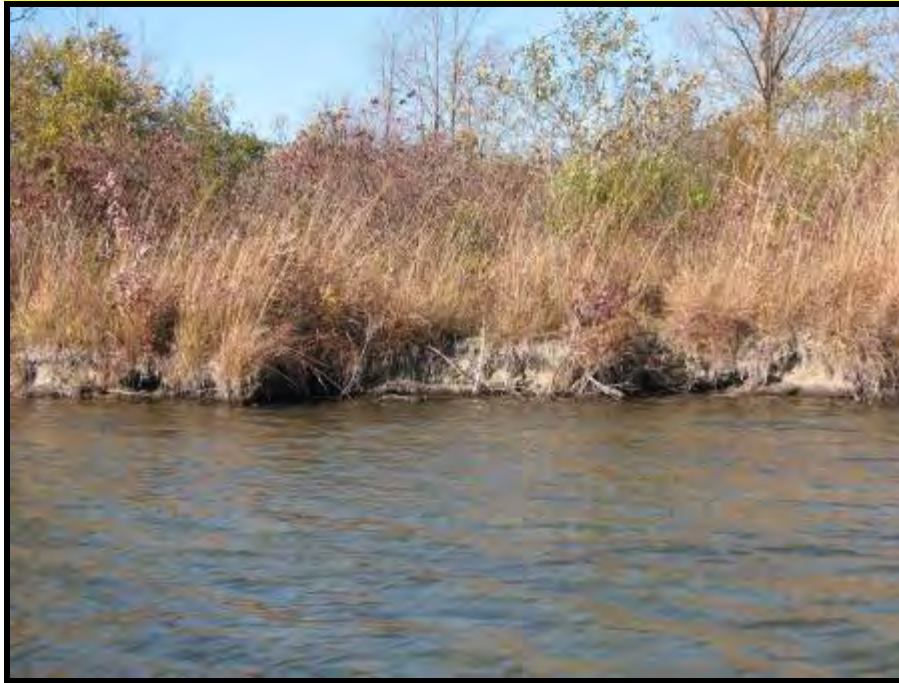
Figure 88. Shoreline erosion occurring at Site 2 on the west side of Oliver Lake.
