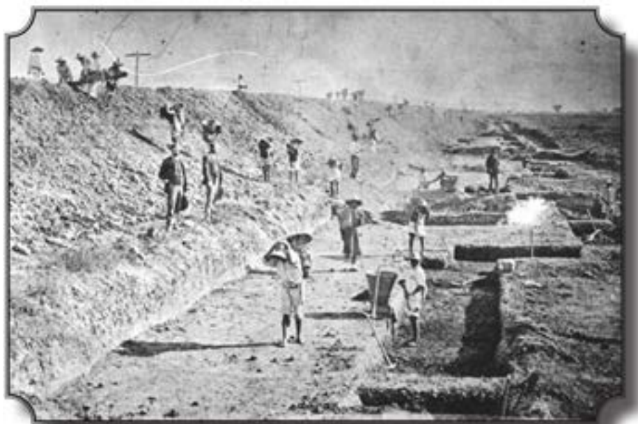
A Southern California railroad construction scene, c. 1880s, shows Chinese laborers removing earth in baskets.
