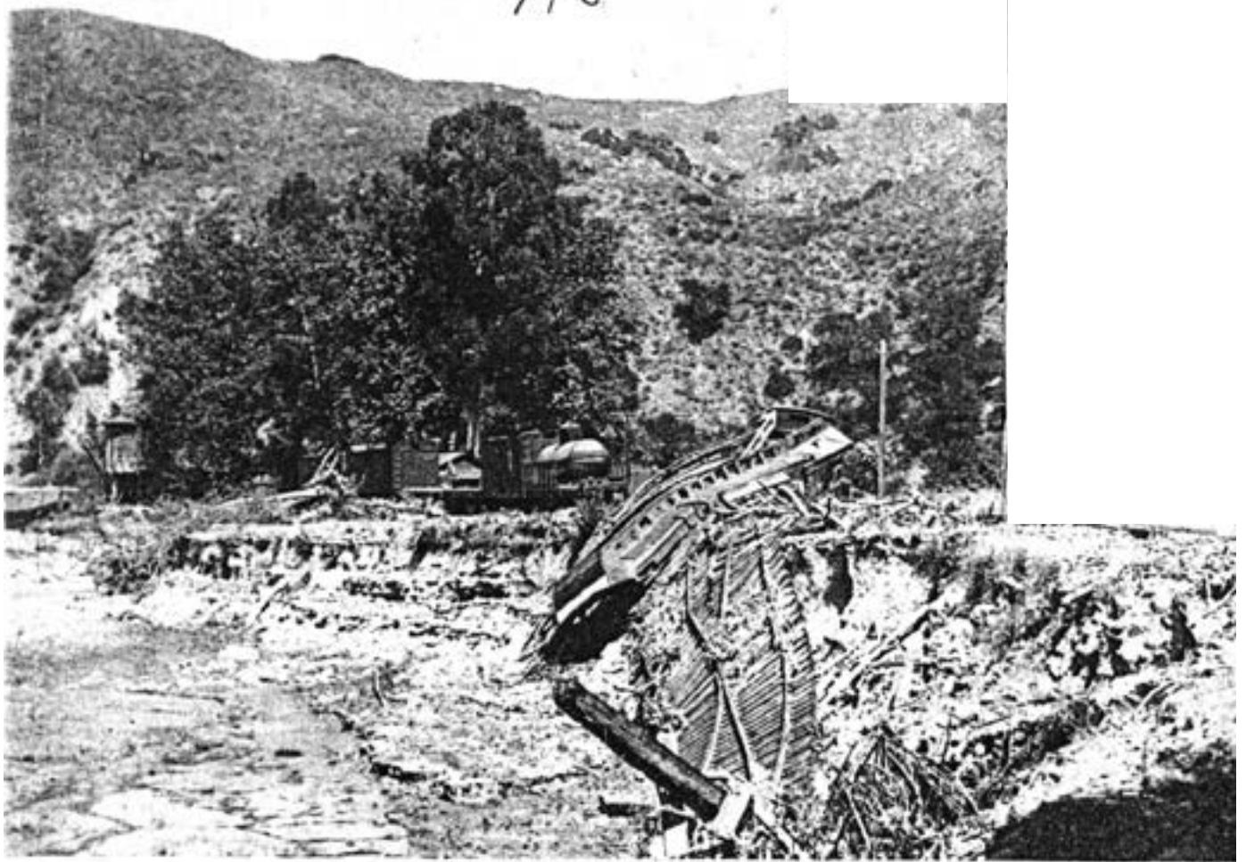
THE BIG FLOOD — In the winter of 1916 a torrent of water rushed down the Temecula Canyon and the Santa Margarita River and washed out the railroad track which ran from Oceanside through Fallbrook to Temecula. The water wash-
