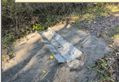
Crossover Dip—Newly Constructed
