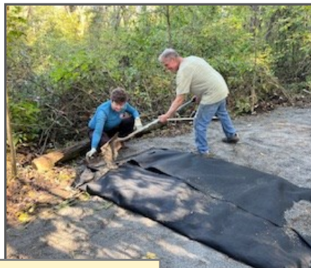
Assembling Trail “Mattress” for Drainage
