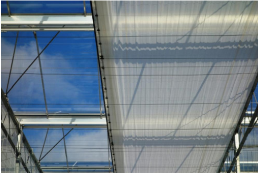
Retractable shade nets can be deployed inside a greenhouse to reduce light intensity.
