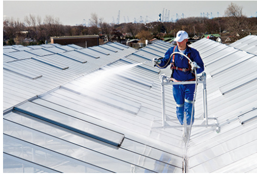
Spray coatings can be applied and removed depending on greenhouse requirements.
