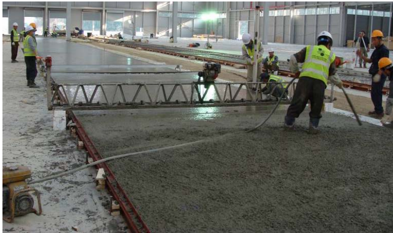
Figure 10: Long strip construction
