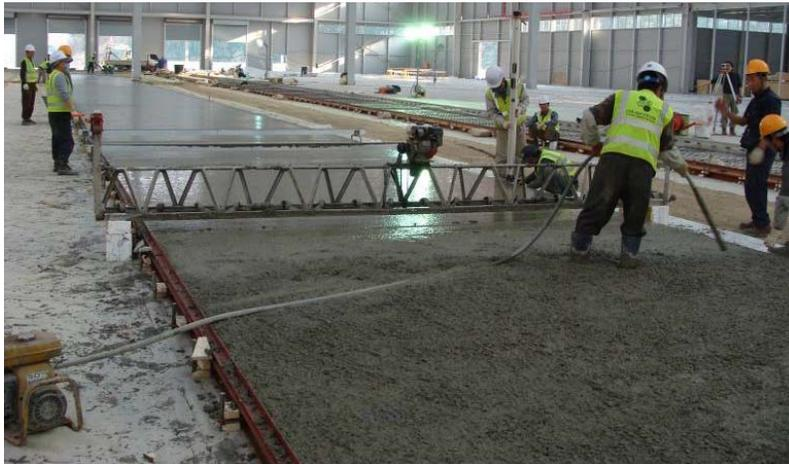
**Figure 10: Long strip construction**
