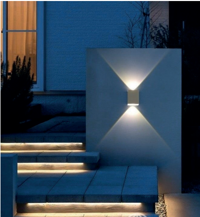
◆ Wall And stair Light
