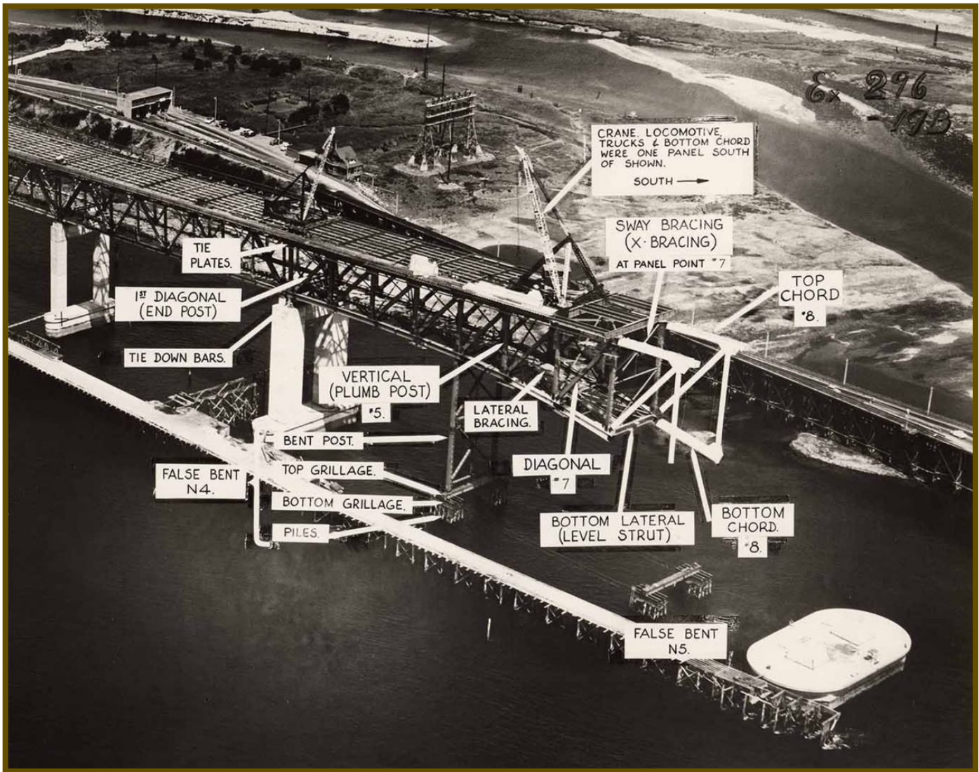
George Allen's photo of Second Narrows Bridge (later Ironworkers' Memorial) over Burrard Inlet, two days before its collapse. Photo by George Allen Air Photos Ltd
