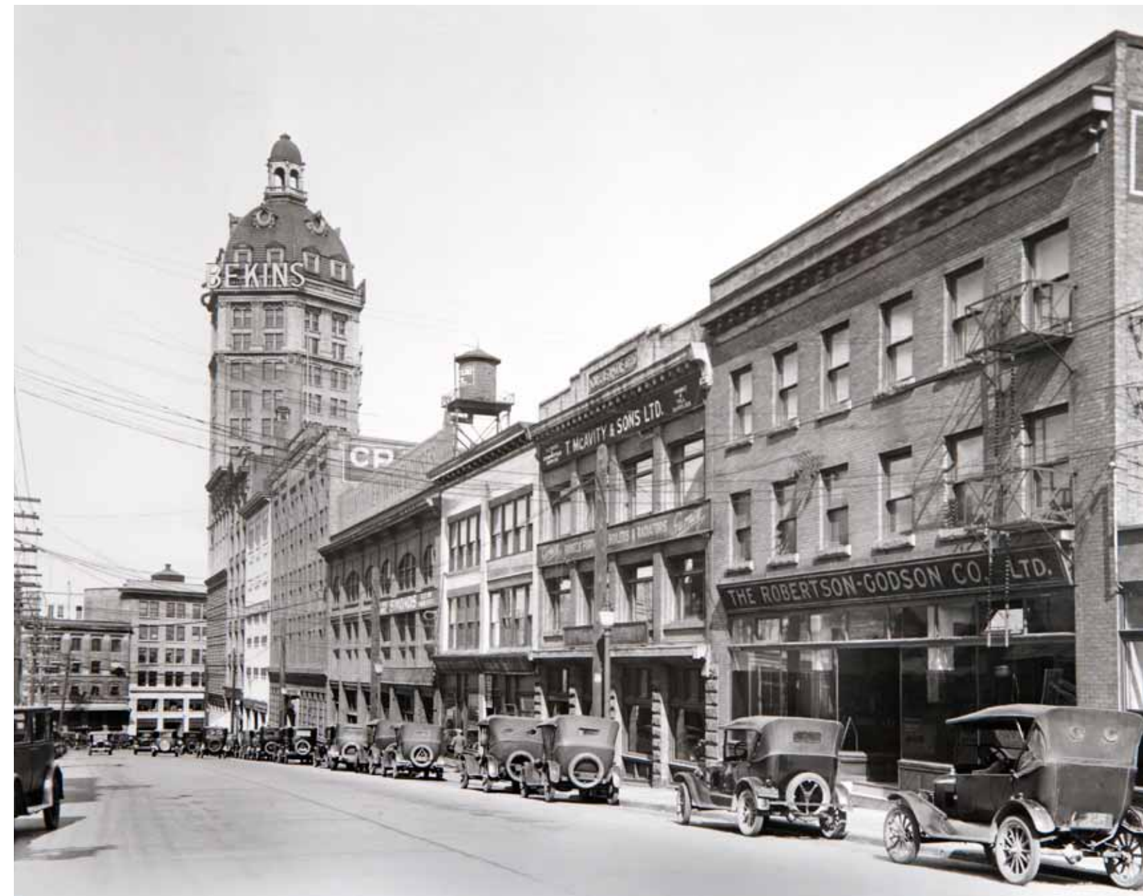
The Robertson-Goodson Co. Ltd., a plumbing supply facility located on Beatty Street south of the Sun Tower and immediately north of the Beatty Street Drill Hall, was the scene of the tragic elevator accident that claimed the life of the Major's son Hugh.
