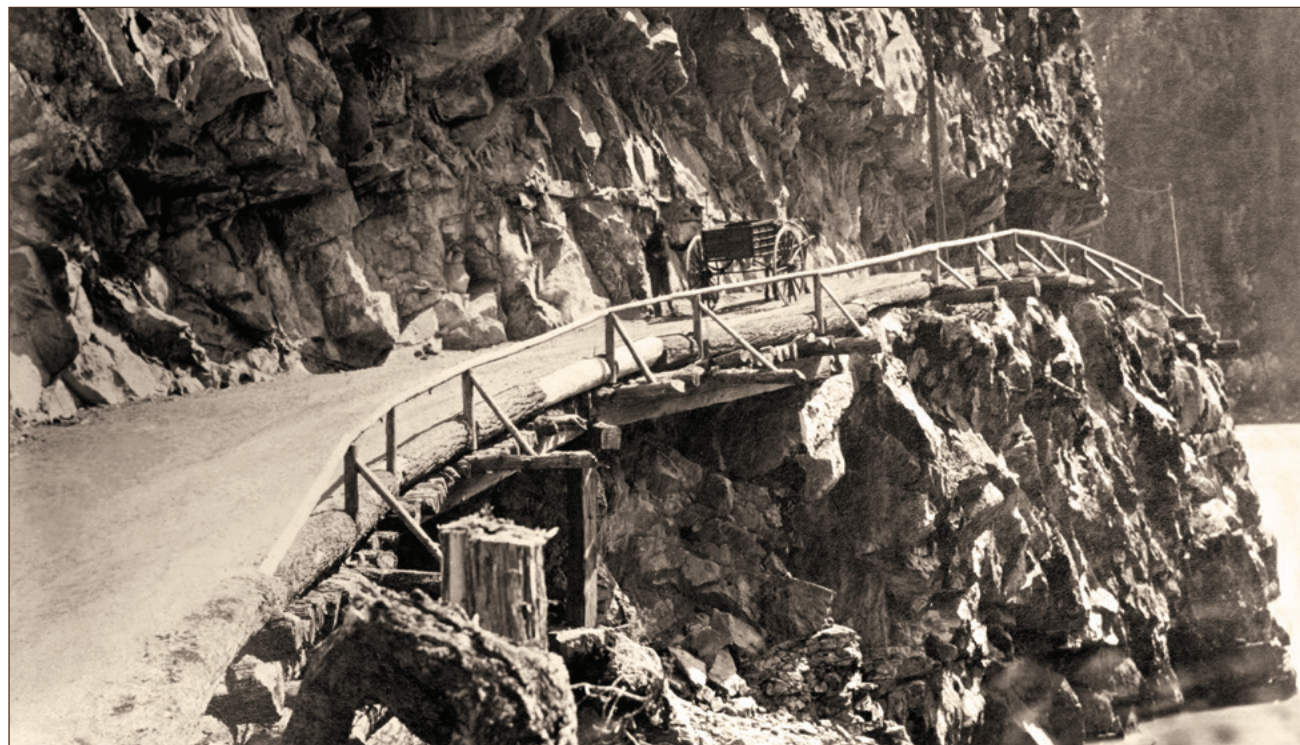
Chapman's Bar Bluff was part of the first 6 mile section of the Cariboo Wagon Road north of Yale that was built by the Royal Engineers between May and November 1862. The road had to be blasted from rock or suspended over the many tributaries into the Fraser River on cribbing and bridges. Note photographer Dally's horse and buggy on the road.
