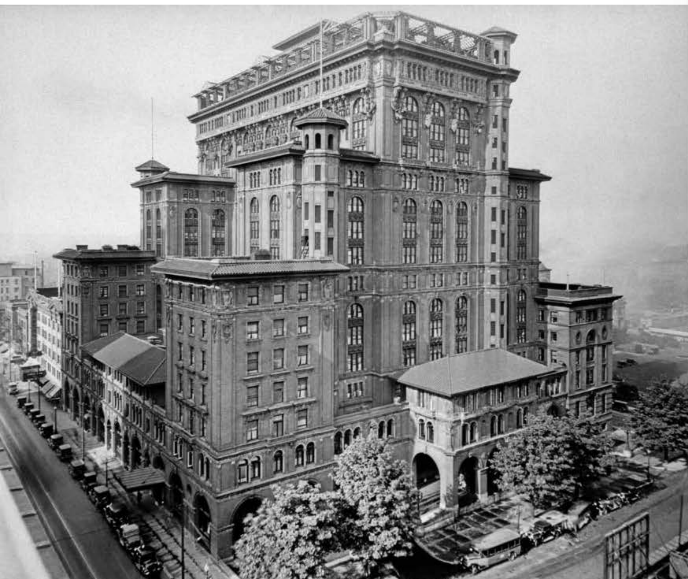
The second CPR Hotel located at the corner of Georgia & Granville Streets.
