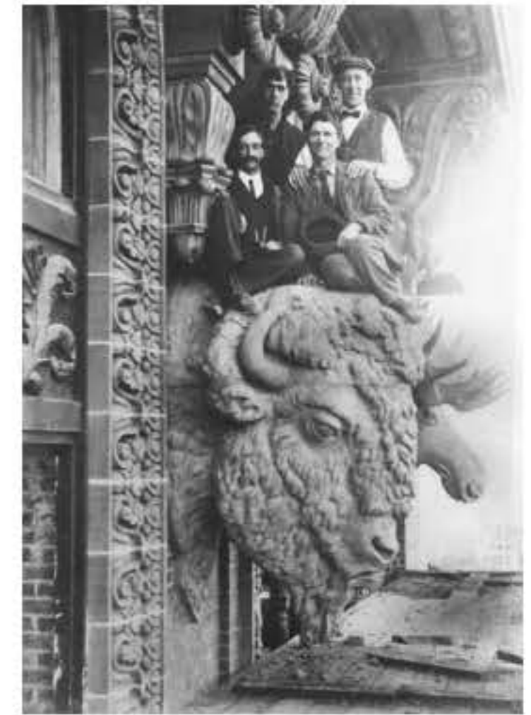
Risk takers pose for a photograph 150 feet above ground during the construction of the second CPR Hotel.
