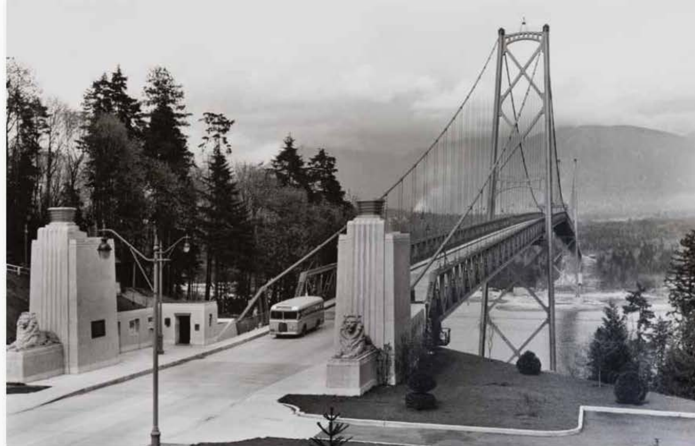
The Entrance to the Lion's Gate Bridge from the Stanley Park side of Burrard Inlet in 1939.
