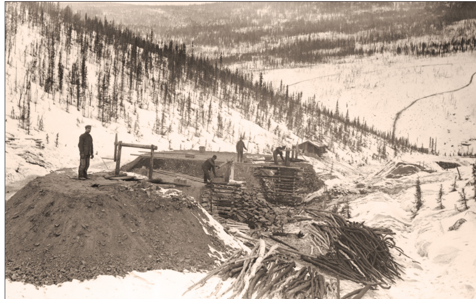
MINERS WORK AT EXCAVATING A SHAFT TO REACH THE PAY DIRT AT BEDROCK. THE MUCK WAS PILLED AROUND THE SHAFT WHILE THE PAY DIRT WAS TAKEN AWAY IN A WHEELBARROW FOR SLUICING IN THE SPRING.
