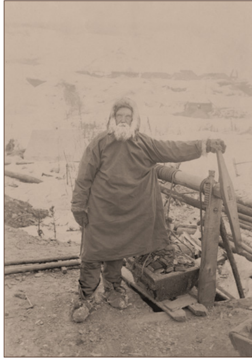
A cold gold miner works at the windlass at 40 below Fahrenheit in the Yukon's valley floor in the winter of 1897-1898.
