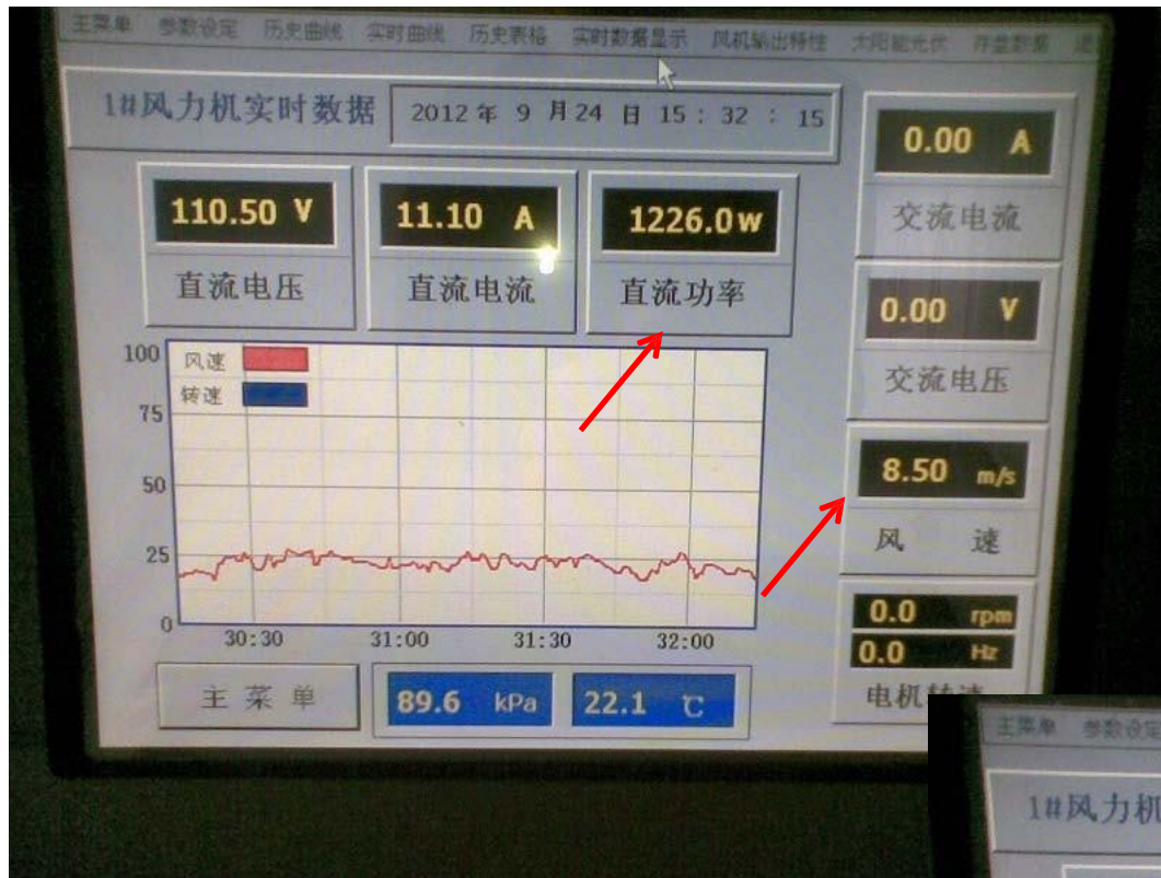
P.11 Real Time Data of Turbine No.1
