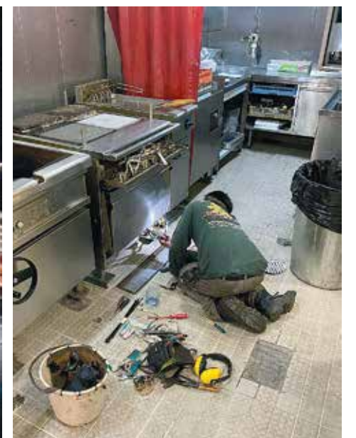
wiring on the galley stove. Pitching in were ERJ Reynato Llona, #3901; REJ Cedric Joseph, #3913; DJU Rey Farinas, #3871 and Wiper Shane Adriano, JM-5345.
