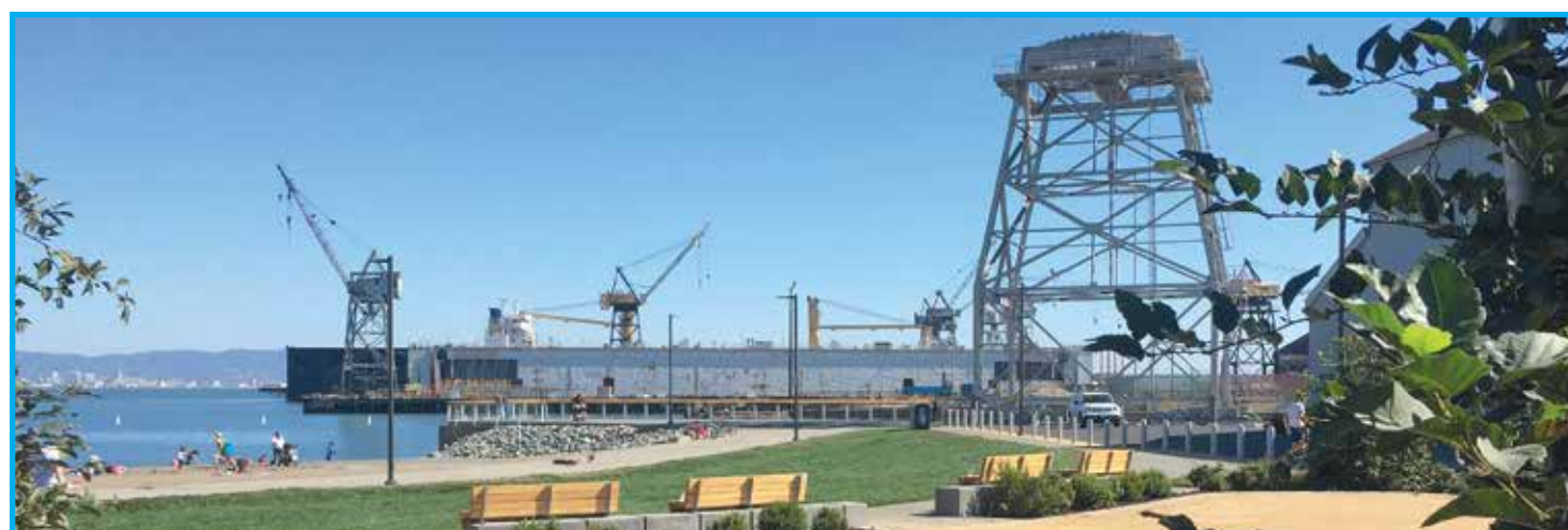
The stack and gear of the CV Kamokuiki (in the background) pictured from Crane Cove Park, a new seven-acre park along the Bay in San Francisco's Dogpatch neighborhood. The new open space pays homage to the city's rich maritime history.
