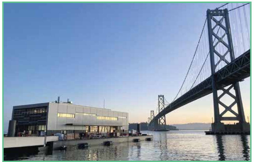
Pictured near the San Francisco-Oakland Bay Bridge is the world's first floating fire station at Pier 22 1/2 in San Francisco (about a half-mile from MFOW Headquarters).
