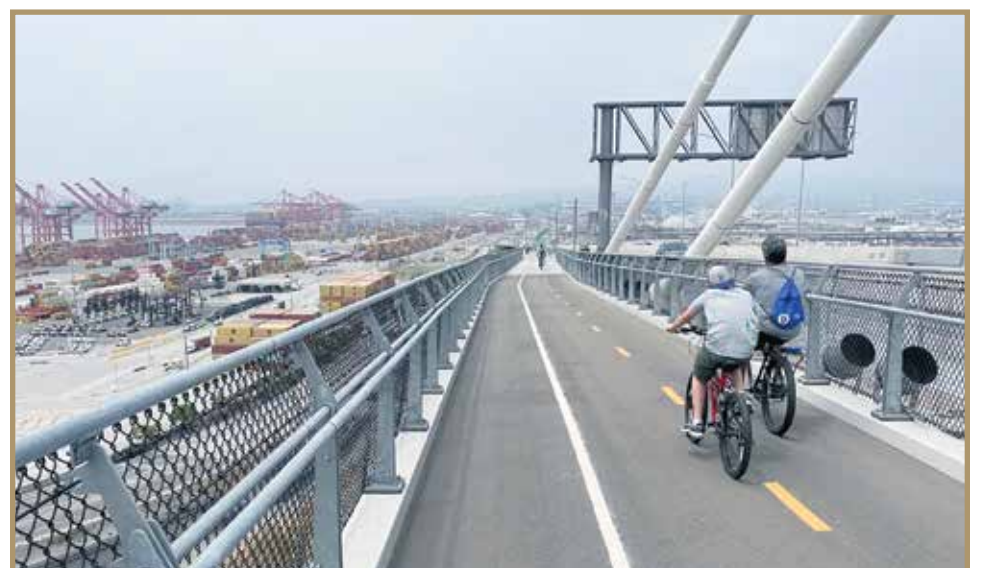
Westbound view on the new Mark Bixby Memorial Bicycle-Pedestrian Path.
