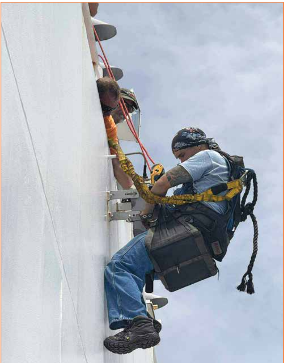
USNS Sisler Electrician Deyne Umphress, #3899, working aloft on helicopter deck lighting system.
