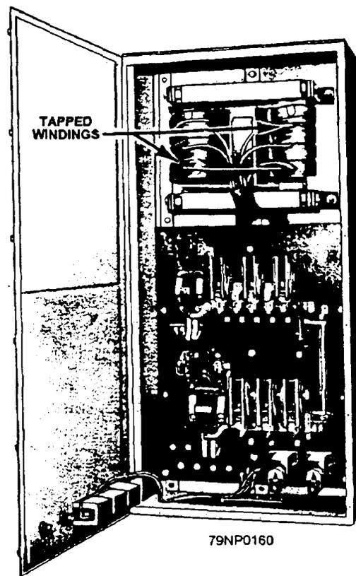
Figure 6-19.—Autotransformer controller.
