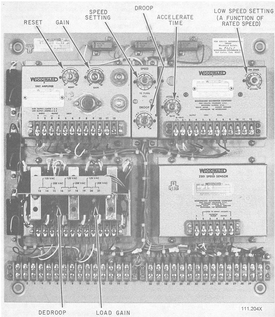
**Figure 9-14.—2301 load - and speed-sensing control.**
