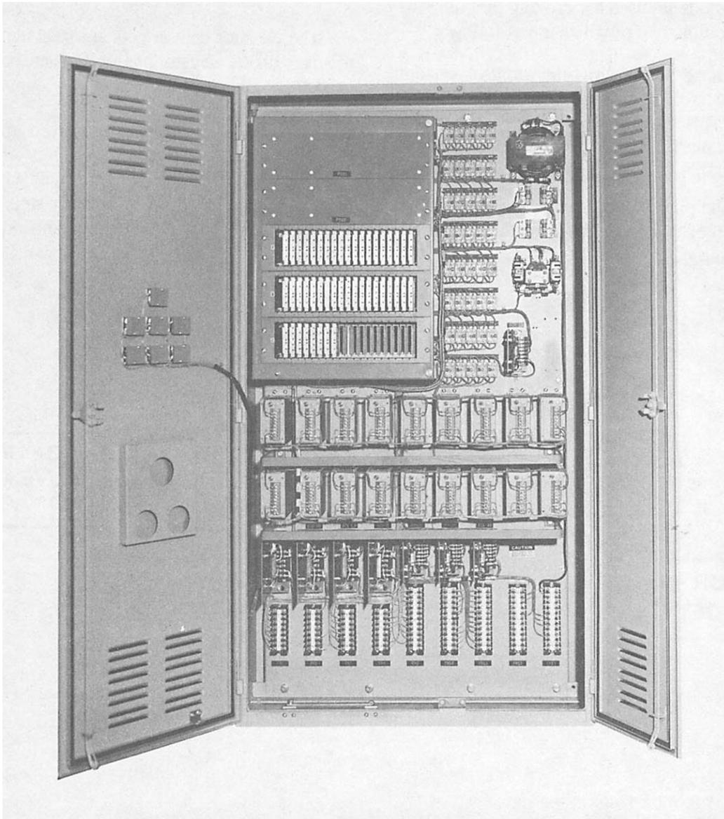
**Figure 5-26.—A static logic panel at the sixth level for a cargo elevator.**
