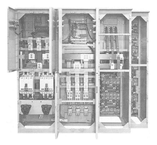
Figure 3-9.—Rear view of a switchboard showing bus bars and disconnect links.
