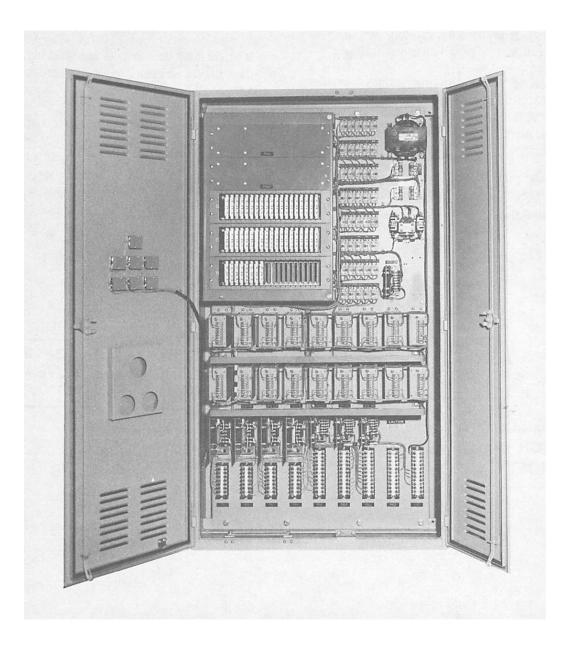
Figure 5-26.—A static logic panel at the sixth level for a cargo elevator.
