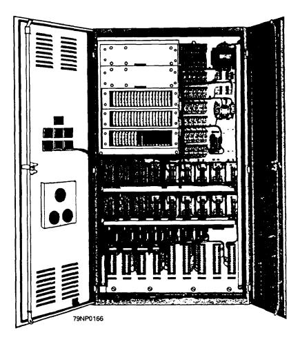
Figure 6-25.—A static logic panel for a cargo elevator.
