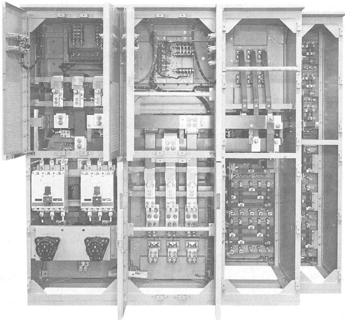
**Figure 3-9.—Rear view of a switchboard showing bus bars and disconnect links.**
