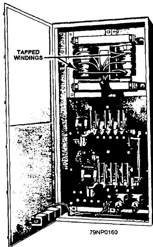
Figure 6-19.—Autotransformer controller.
