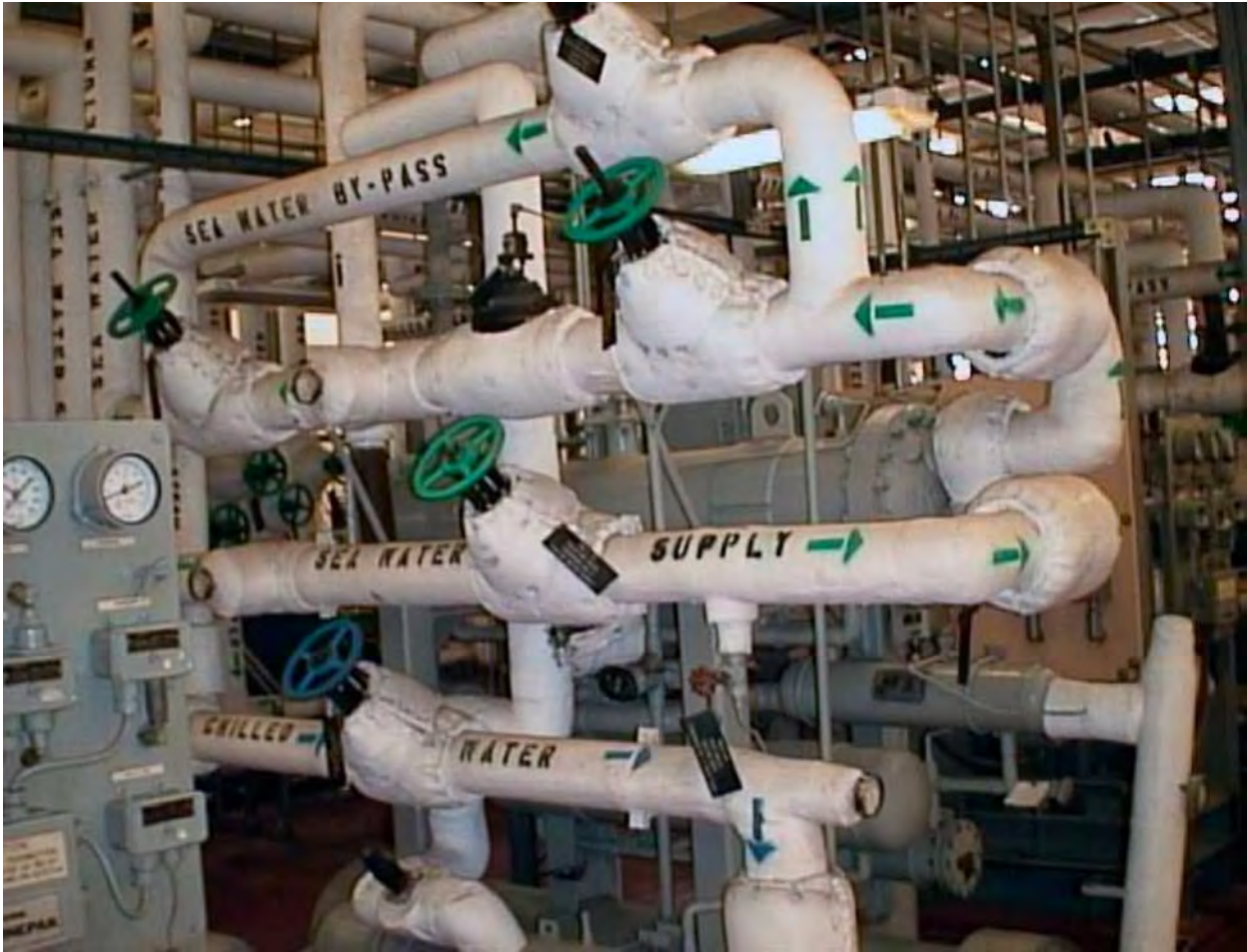
Figure 5-1- Piping directional flow.
