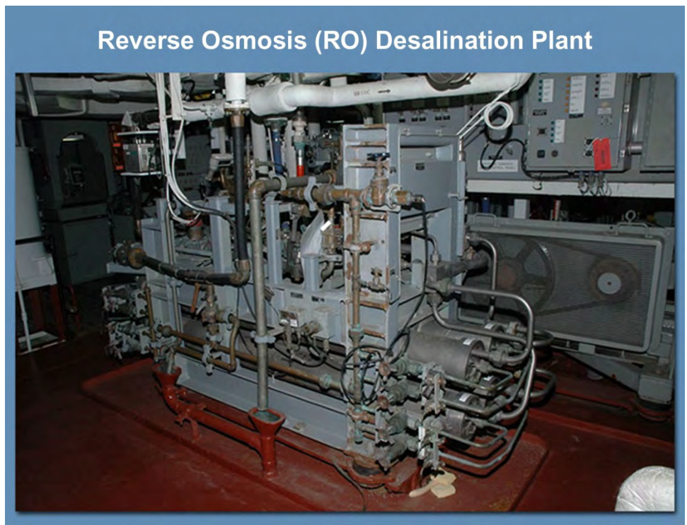
Figure 18-13 — Reverse osmosis (RO) desalination plant.
