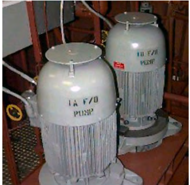
Figure 12-5 — Fuel oil (FO) service pump.
