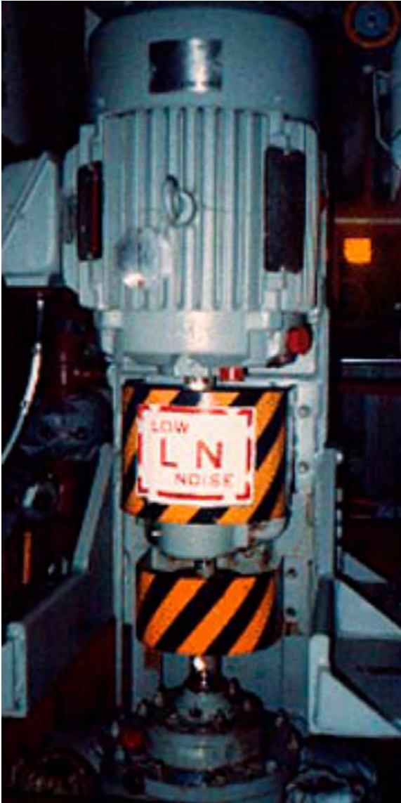
Figure 12-6 — Fuel oil (FO) transfer pump.
