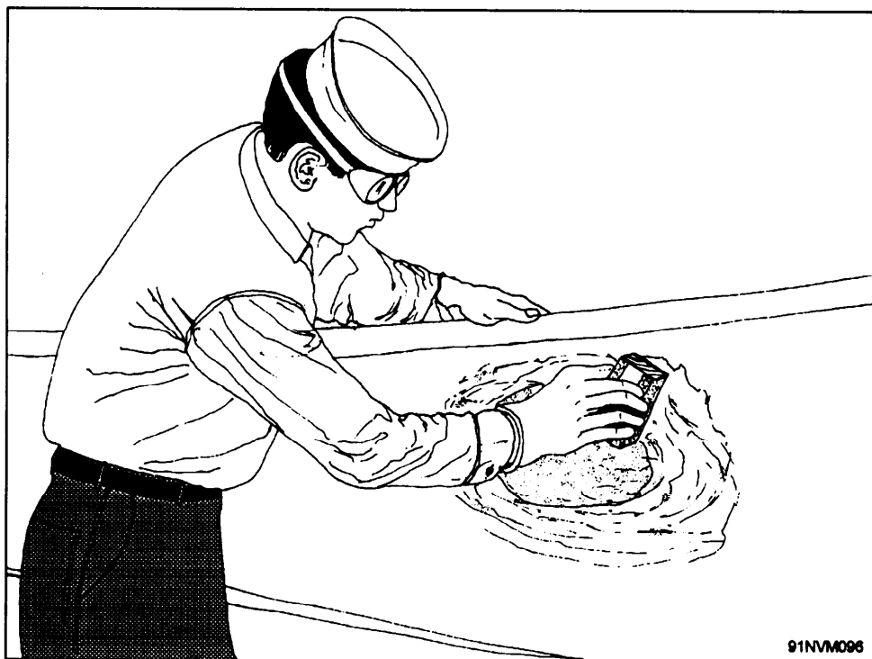
Figure 4-16.—Sanding a completed patch.
