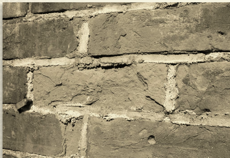
This photo shows brick damage caused by using modern mortar on older soft bricks.
