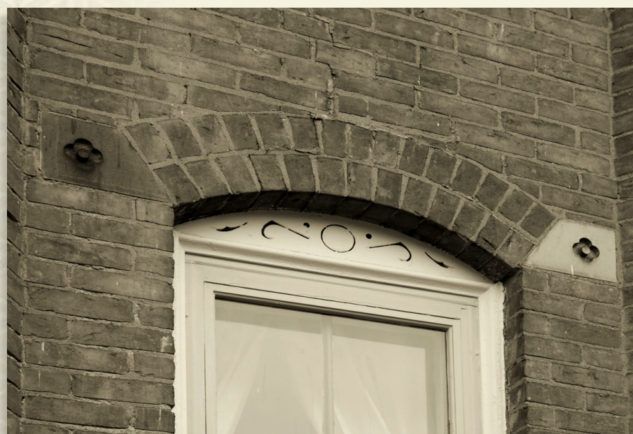
Masonry details such as an arched header over a door or window opening are common. Also note the limestone blocks at either end of the arch.
