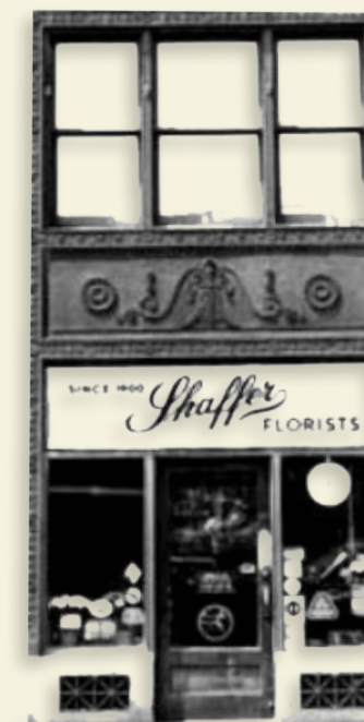
This finely detailed bronze storefront is typical of many constructed during the 1920s. The original grilles, spandrel panel, and windows are all intact.
