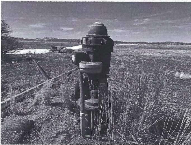
LEFT: 40 HP pump and well that services the irrigated cropland
