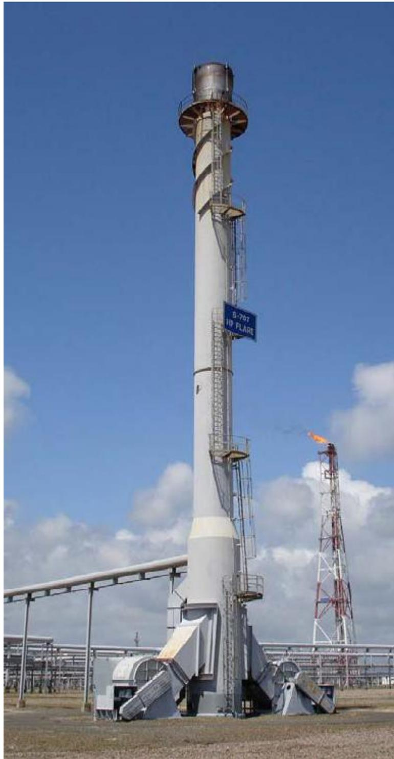
A gas flare, alternatively known as a flare stack or tower is used to eliminate waste gas which is otherwise not feasible to use or transport. They also act as safety systems for non-waste gas and is released via pressure relief valve when needed to ease the strain on equipment
