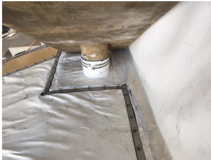
Figure 1. Photographs of mechanical attachments and pipe boot.
