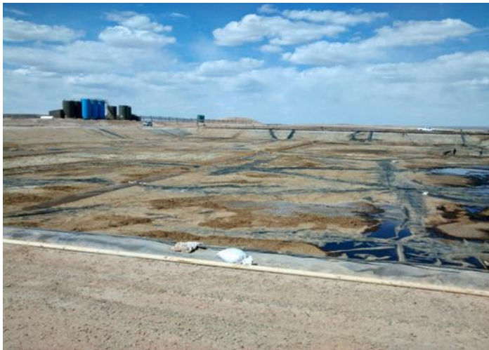
Wyoming - Sediment in pond bottom after removal of water for primary geomembrane repairs; pond operational for seven years before repairs.
