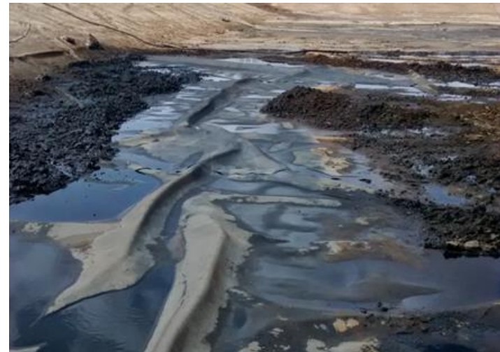
Sediments removed carefully by hand using plastic shovels and low-pressure power washer, then wheelbarrowing the sediments to the top of the pond.
