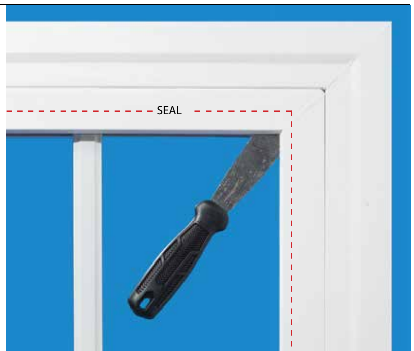
ACCESS FOR PUTTY KNIFE ON EXTERIOR
