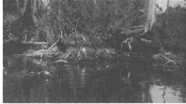
FIG. 5. Closer view of the base of the cypress "island" in Figure 4, showing the exposed roots of the cypresses and bay shrubs and the general aspect of degradation.
