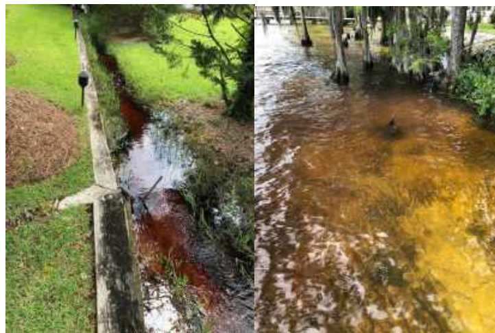
Figure 13. Left photo shows the NC DOT drainage ditch at 580 White Lake Drive after a rainfall event; right photo taken at the lakeshore at the same location, on the same date (June 27, 2018). Total rainfall for the month of June 2018 was 10 inches (Table 2).
