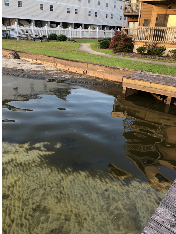
West side of the lake, June 15, 2022
