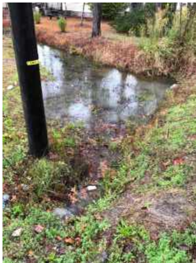
Figure N6. Stormwater ditch behind Bladen Medical Center at White Lake Drive and Lennondale Road, after the same three-inch rain, February 7, 2020. Note the cloudy appearance of the water.
