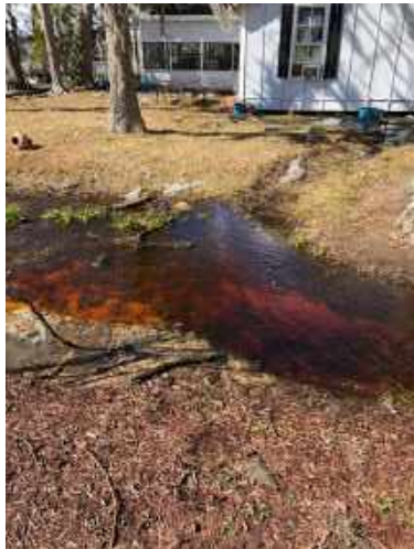
Figure N7. Views of the NC DOT drainage ditch at 408 White Lake Drive on February 7, 2020. Residents on either side of the ditch are also draining their yards into the ditch (photo on bottom). This ditch is closer to (and connected to) the drainage area behind the Bladen Medical Center.
