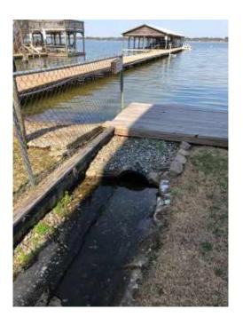
Because lake levels are so high now, there is backflow from the lake into stormwater outfalls. Much debris can be observed in shallow areas of the lake, which is what most property owners are seeing.
