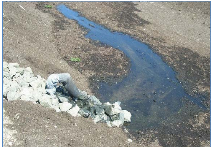
Sock filter used to remove solids prior to water disposal (OR)
