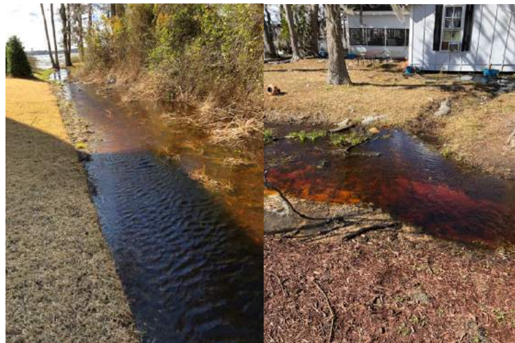
Figure N5. Views of the NC DOT drainage ditch at 408 White Lake Drive on February 7, 2020. Residents on either side of the ditch are also draining their yards into the ditch (photo on right). This ditch is closer to (and connected to) the drainage area behind the Bladen Medical Center.
