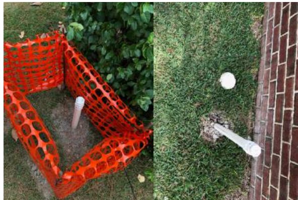
Figure N2. Top photo: groundwater well at Timberlodge Lane, located in a landscaped island that is popular with dogs—the fencing was added by Town staff when they rehabbed the well. Bottom photo: groundwater well at Godwin Road that was also rehabbed by Town staff. The top pipe is a wastewater
