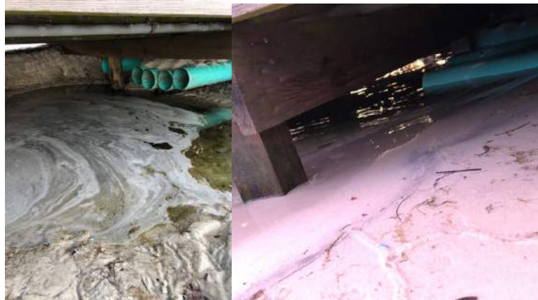
Figure N7. Stormwater pipes under Nathan’s Cove pier: left photo taken October 23, 2019 and right photo taken on February 13, 2020. Runoff is from an asphalt street/parking area for the condominiums.
