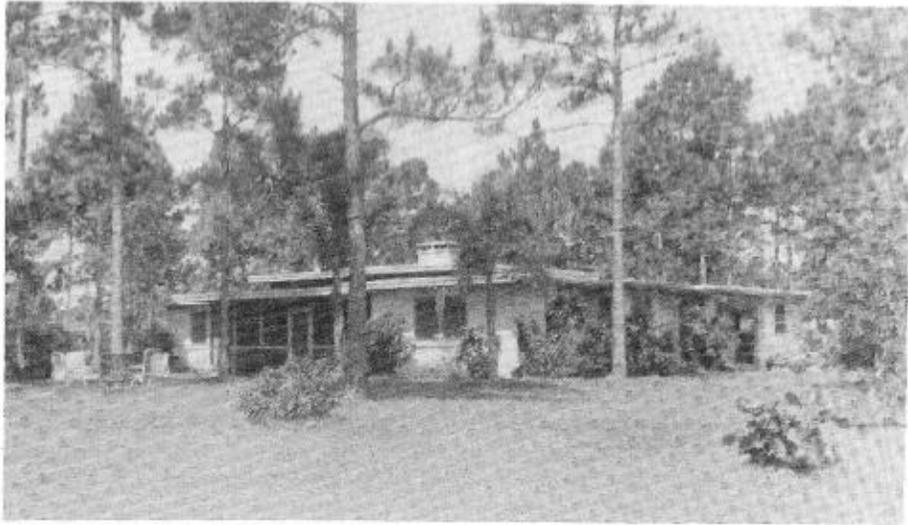
The Ross Home near the Hammock. This home illustrates the unique village architecture. Note the clerestory window at the roofline. The house is angled to the wind, eliminating the need for air conditioning.
