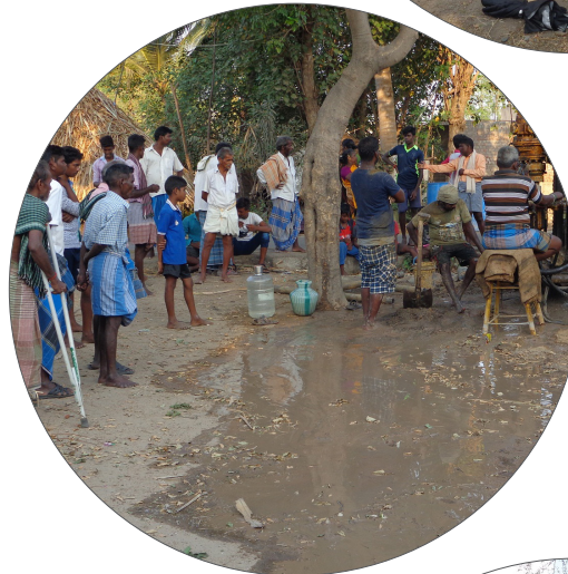
Digging the Borewell
