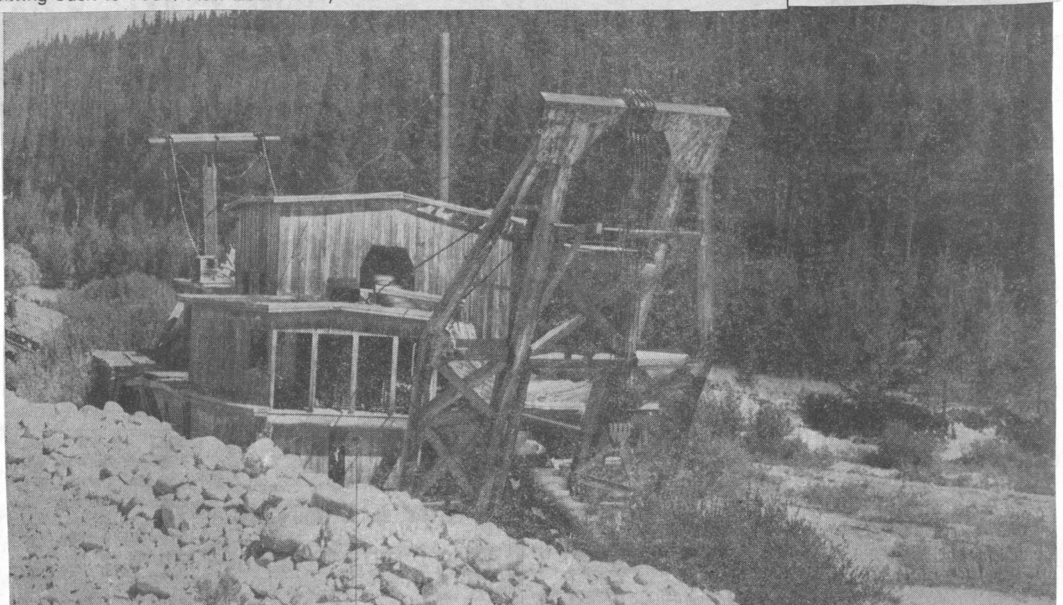
Dredging operations along Steamboat Creek and Warren Creek in the 1930's and early 1940's are recalled by this partly-sunken abandoned dredge, which received electrical power from an Elk Creek power plant.
