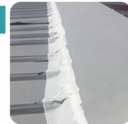
• The overlap between the light steel roof and color steel plate and the daylighting board and the sealing of the joint of the gutter.
