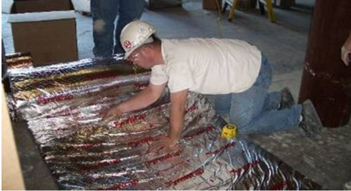
1. Roll out and cut required length of Fyrewrap Elite®.
