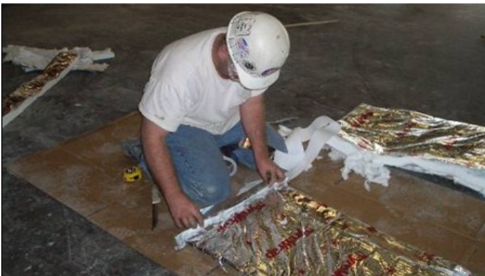
2. Seal all cut edges with aluminum foil tape.
