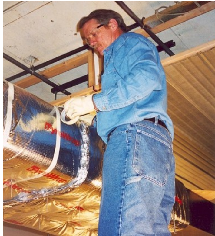
5. Fix material in place steel bands and/or pins where needed.
