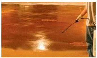
An easy Lp sprayer application Spray apply Pro-Seal DP-36 to wet or pre wetted concrete floors, walls, ceilings, columns, tanks, or other concrete surfaces.
