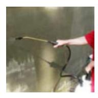
The Green Pro-Seal DP-36 deep penetrating extractant material is spray applied to a pre tap water wetted concrete surface with a hand pump sprayer or an airless system at less than 100 psi. Pro-Seal DP-36 will extract fluid contaminants as it cures and dries out the target concrete substrate, preparing the concrete substrate to receive paint coatings and other wear surface coverings.
