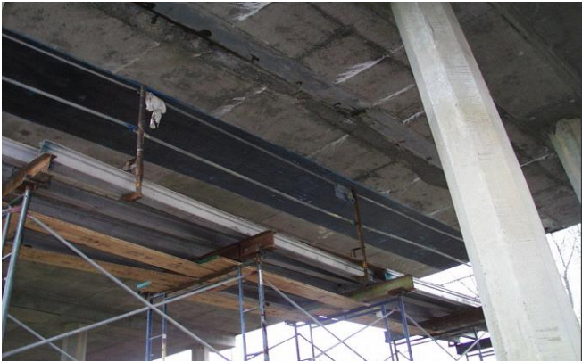
Saddle Strapping to increase structural values
