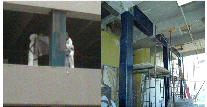
Interior and exterior column reinforcement to recapture and maintain structural values
