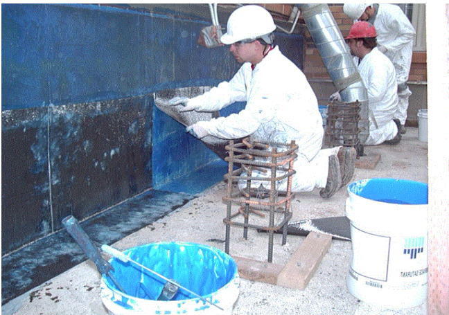
Wall reinforcement to recapture and retain structural values
