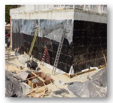
The photo above is an example of an inverted installation of the **Pro-Seal® FlexSystem II Methane Barrier, Waterproofing, and Water Management System™** that will have concrete poured or shot to it.
