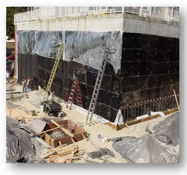
The photo above is an example of an inverted installation of the **Pro-Seal<sup>®</sup> FlexSystem II Waterproofing, and Water and Vapor Management System™** that will have concrete poured or shot to it.
