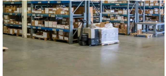
Light duty warehouse Floors
